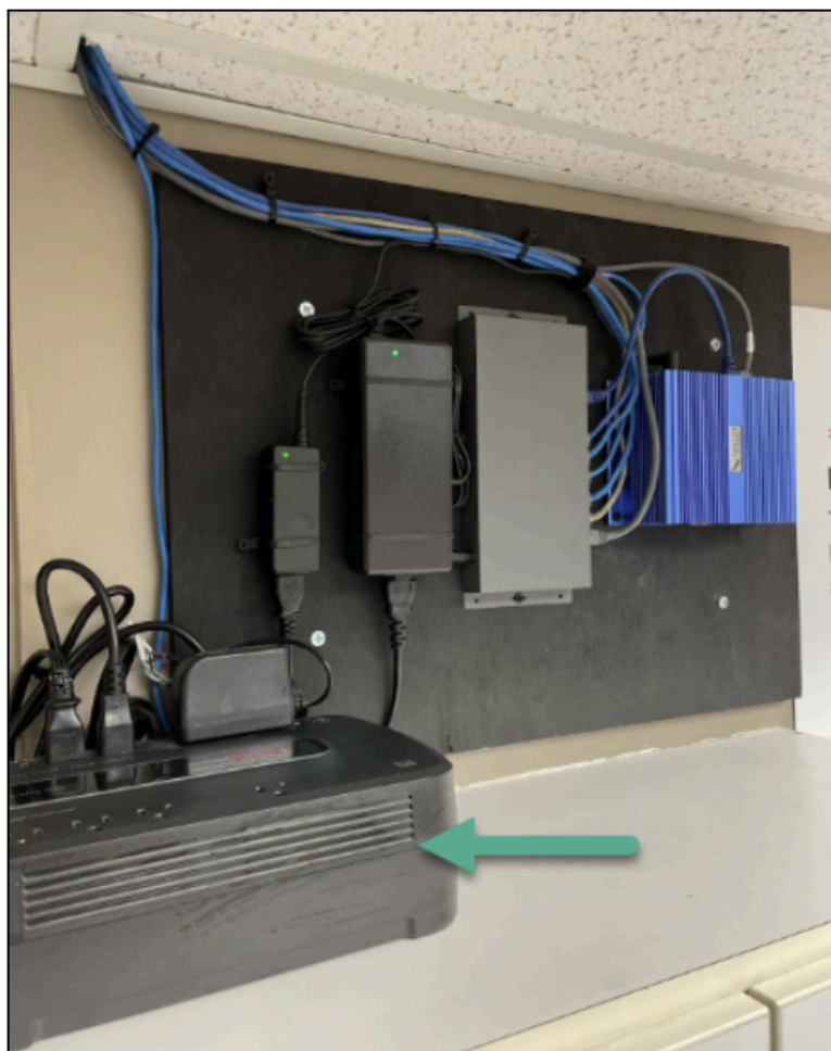
GOOD EXAMPLE: A Bridge mounted with painted plywood (nice touch) with clean cables and securely fastened hardware. Note the UPS power solution.
