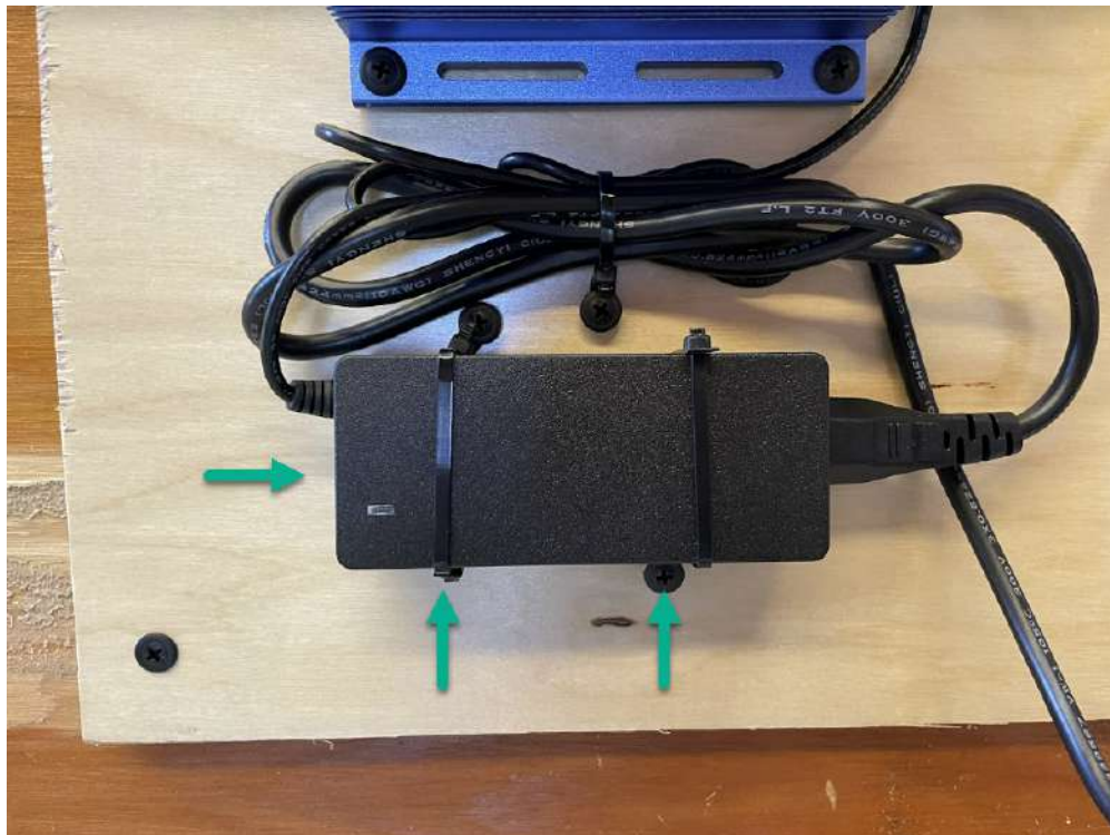
GOOD EXAMPLE: Do securely mount the power supply using zip ties and screws to prevent cords from accidentally falling out.
